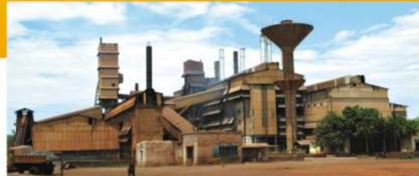
Ferro Chrome Plant at Garividi
