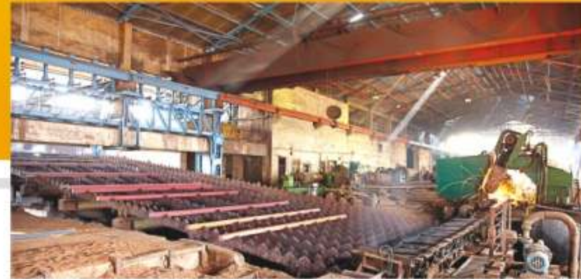
Turnover Cooling Bed at Facor Steels Ltd., Nagpur
